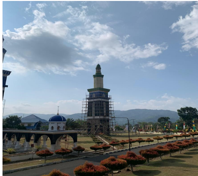
Figure 5: Rehabilitated tower Source: Researcher Documentation, 2024
