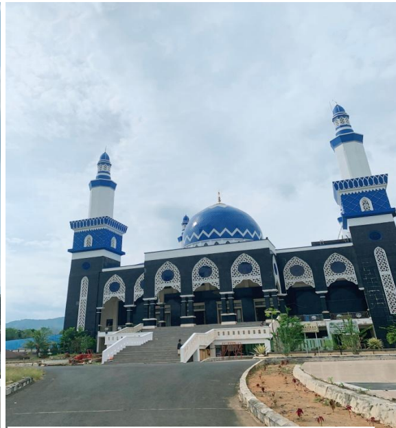
Figure 7: Rear view of the mosque after repainting
